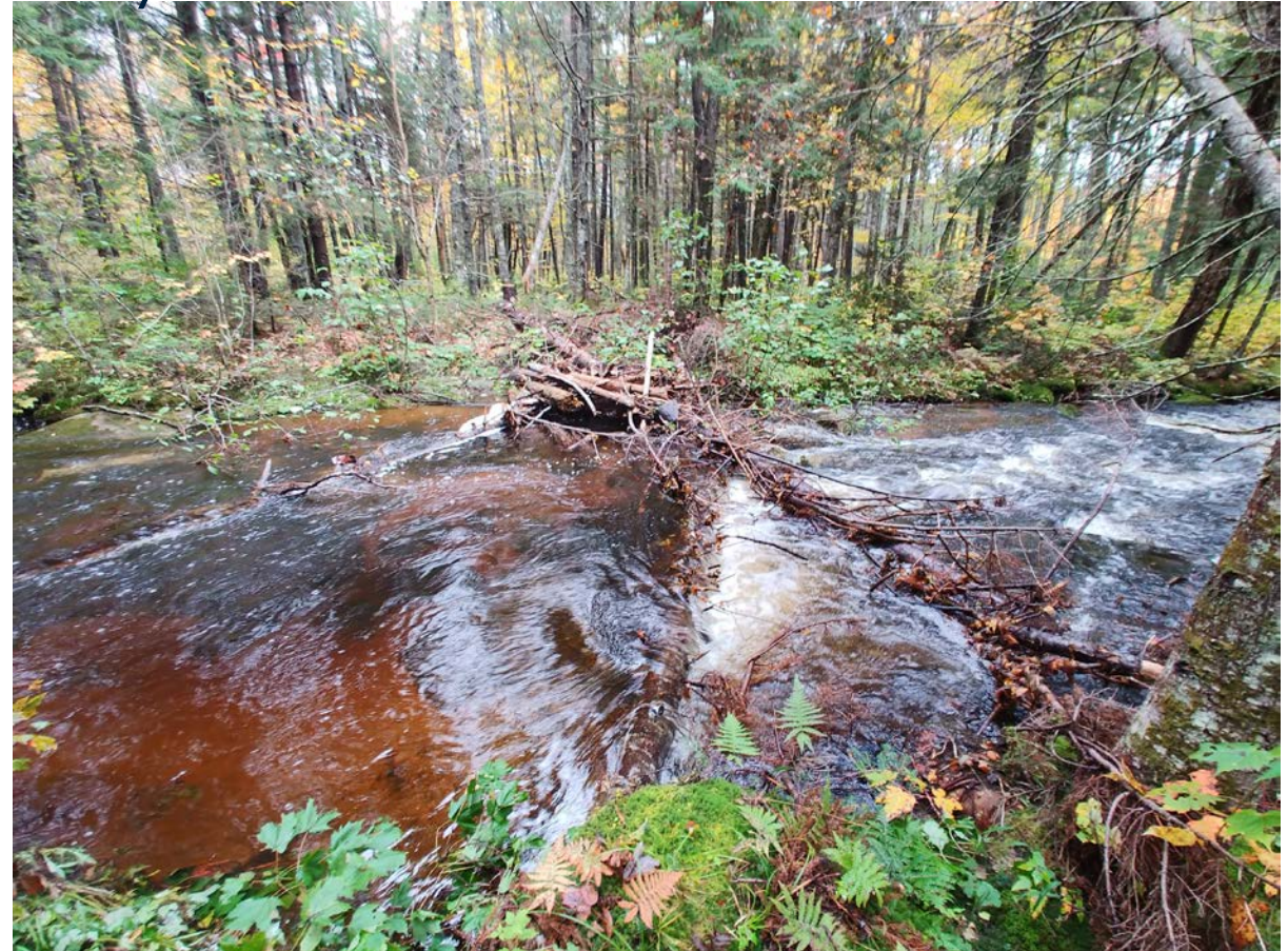
One year after installation
