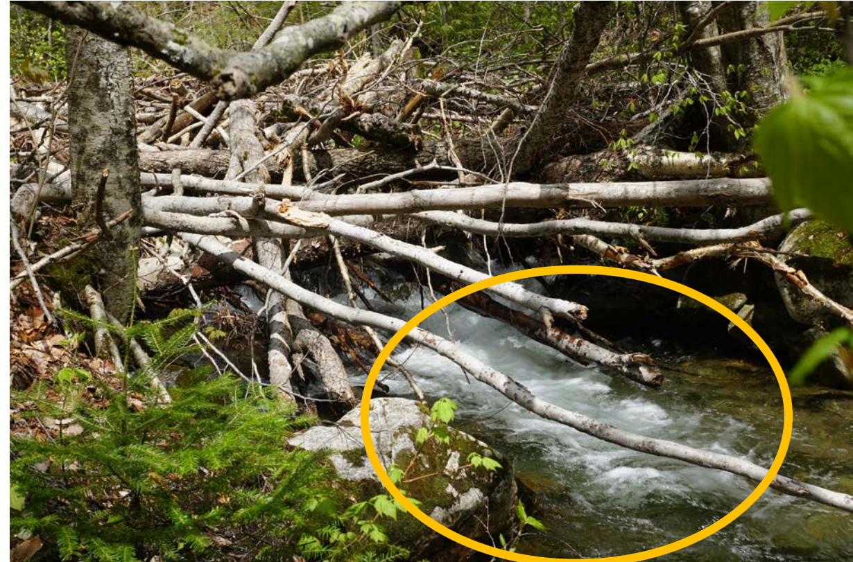
New scour pool, +4' deep
