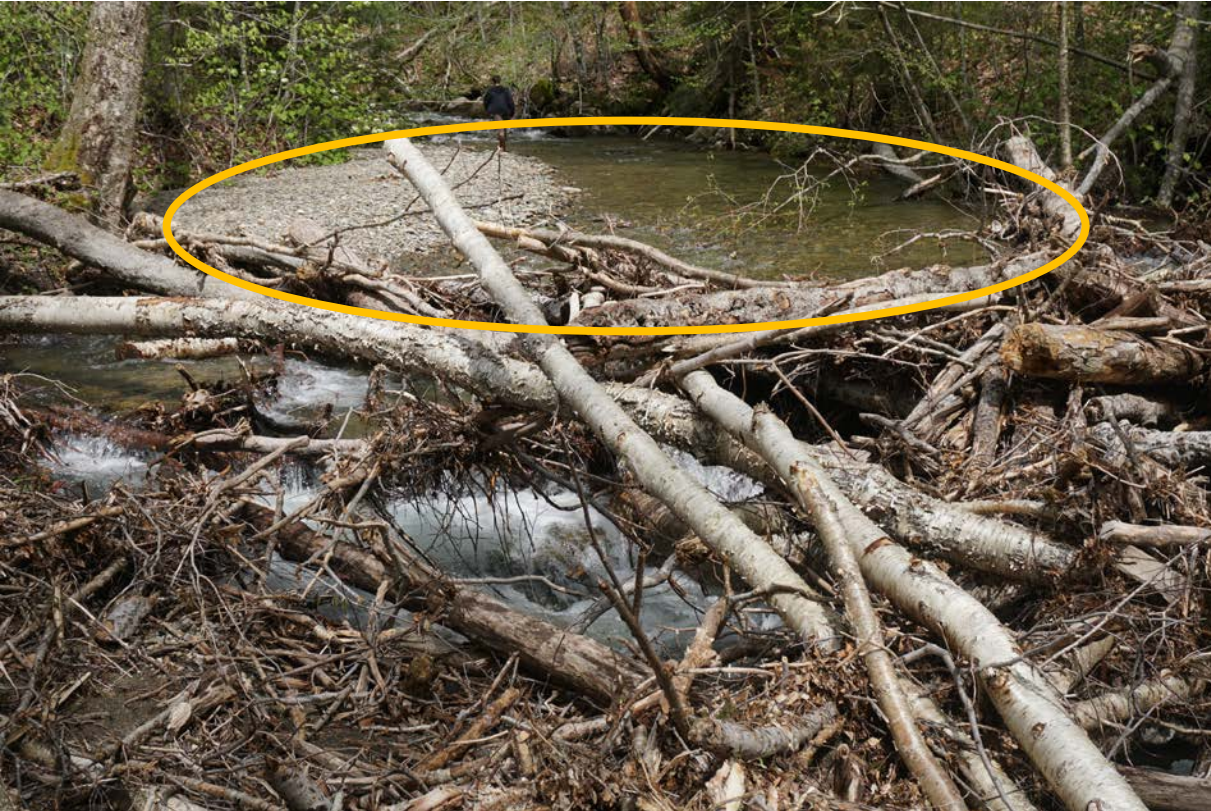
Aggraded gravels and cobbles raised bed several inches
